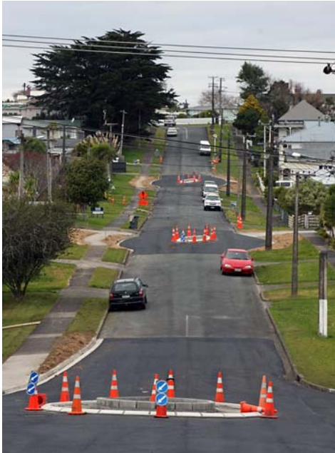
• The road works underway in Puriri Street
