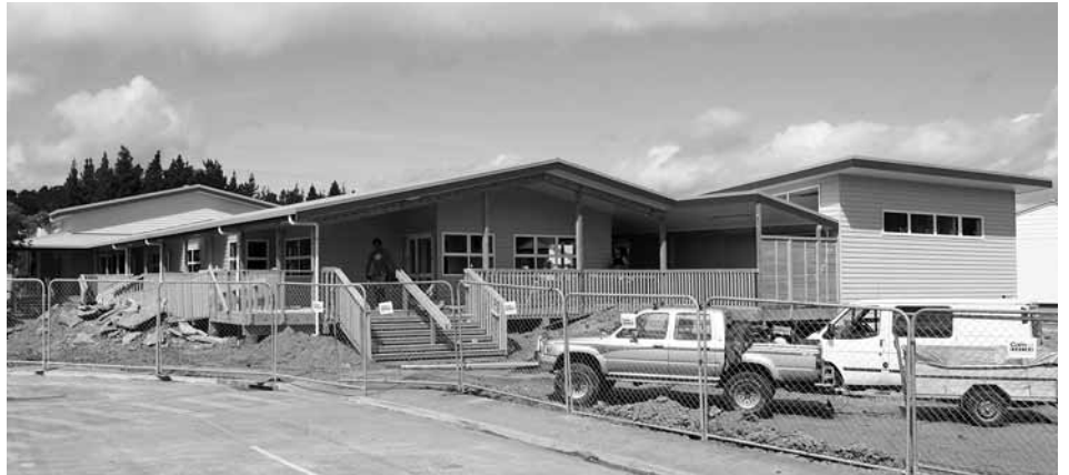
• Builders finishing off the new reception and administration end of the building
