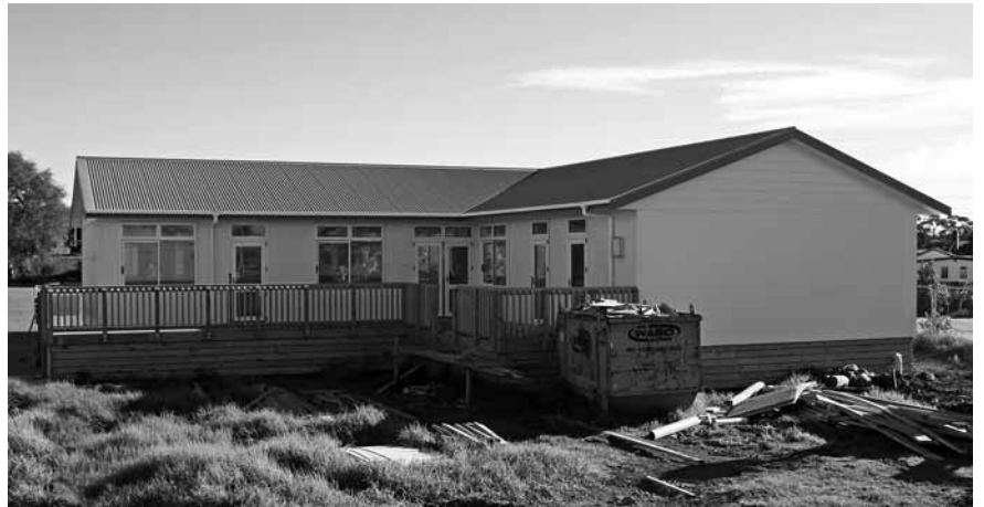
• The almost finished new library and resource building
