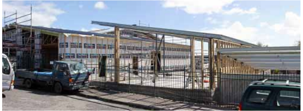
• Work progresses on the new college buildings, seen here from Rautawhiri Rd
