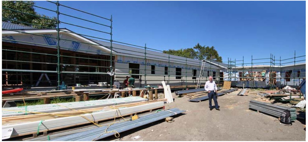
• Craigweil operations manager Richard Parker on the construction site, with the new hospital behind
