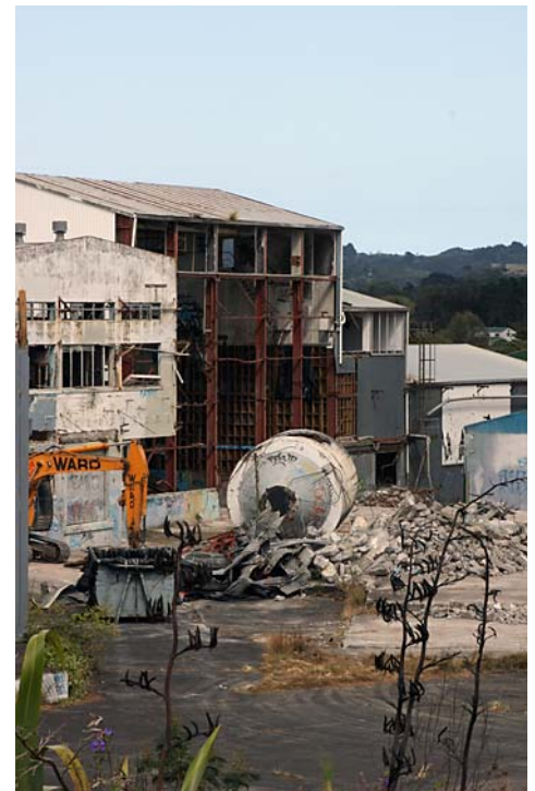
• Demolition work underway on the old dairy company buildings
