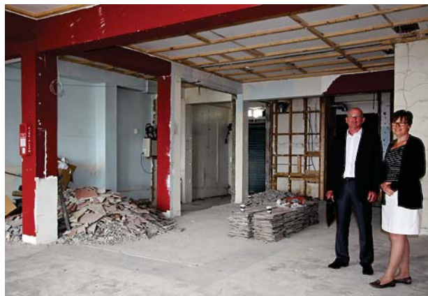
• Alistair and Karen Watts inside the rubble-filled shell of what will soon be the Helensville Pita Pit
