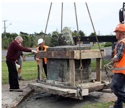
• Laurence McLeod (left) and contractors prepare to lower the cairn onto its new site
