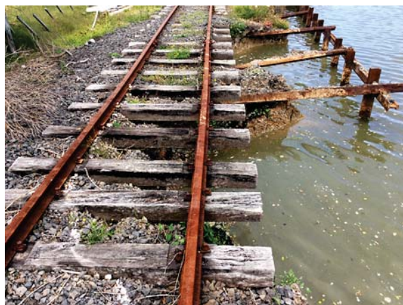
• The washed-out section of the rail triangle
