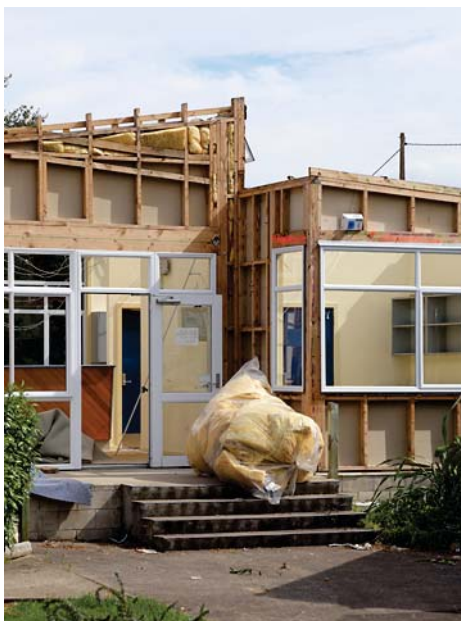
• Demolition work underway on the leaky buildings
