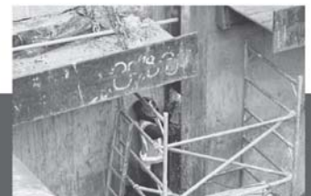
Onsite welding in New Lynn Railway trench.
