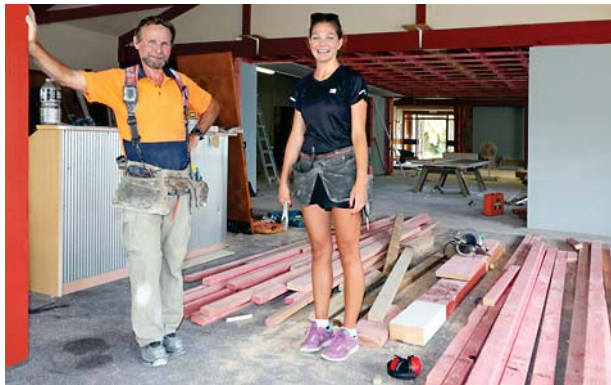
• Electrician Nick Honeycombe and helper Grace Fletcher at the building site
