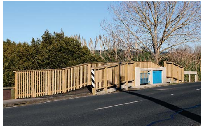
• The new Parakai footbridge railings
