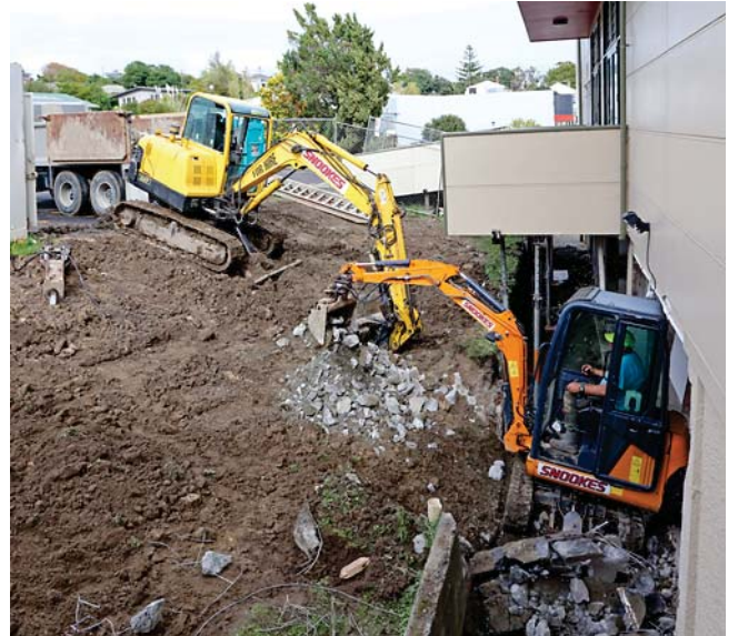
• Excavators prepare for the ramps into the basement
