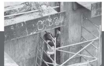
Onsite welding in New Lynn Railway trench.
