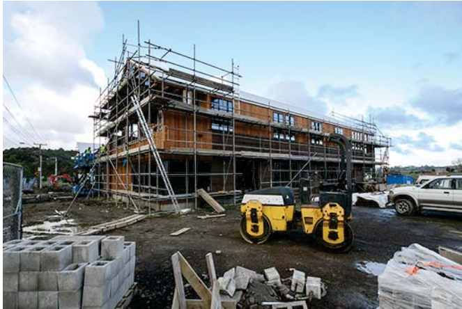
• Building is well underway on the Stage 1 shops and apartments
