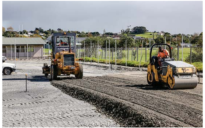
• Work progressing on resurfacing the netball courts
