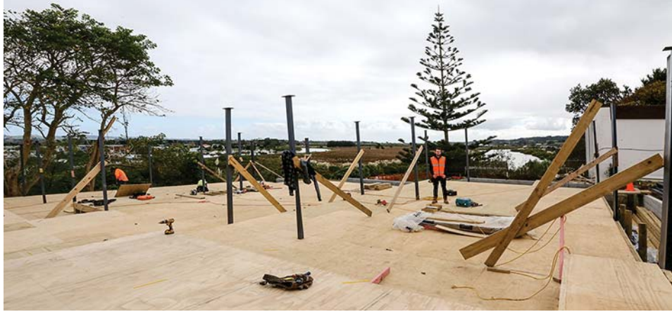
• Rory O'Connor on the building site in Commercial Road
