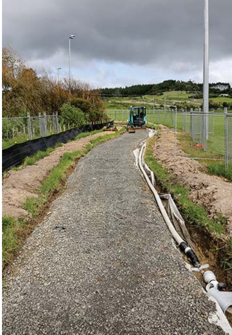
• The new walkway in preparation for concreting
