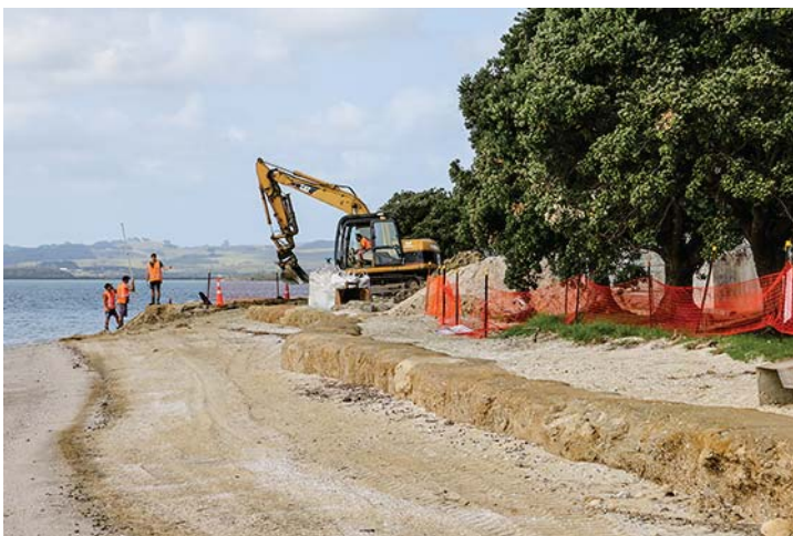
• Work underway on the new 'natural sandstone' seawall
