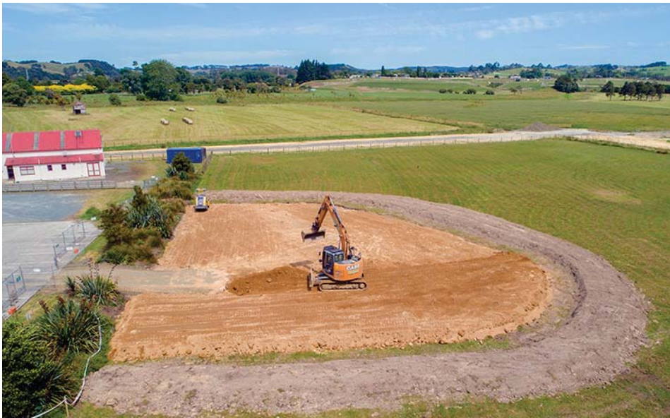
• A digger levels some of the 1000m 3 of soil on the playground site in January
