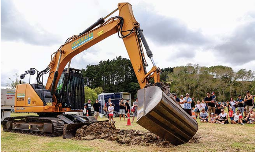
• Above: Heavy machinery at work - a stump pulling operation was a crowd pleaser
