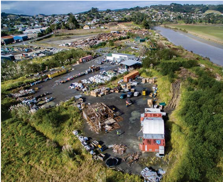
• An aerial view of the Helensville Community Recycling Centre site
