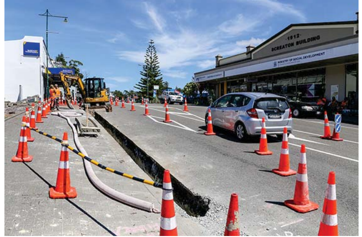
• Excavation work was an early step in the beautification project
