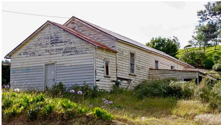
• A dilapidated Woodhill Hall in 2013
