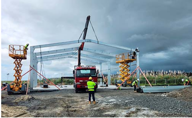
• Framing goes up on the new Rescue Centre building
