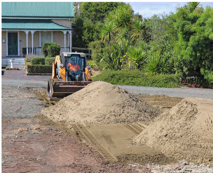
• Dave Swale spreading out sand as a base for the metal
